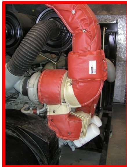
Fabricated cover for turbo-charger and exhaust system piping.
